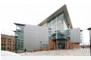
The Bridgewater Hall
